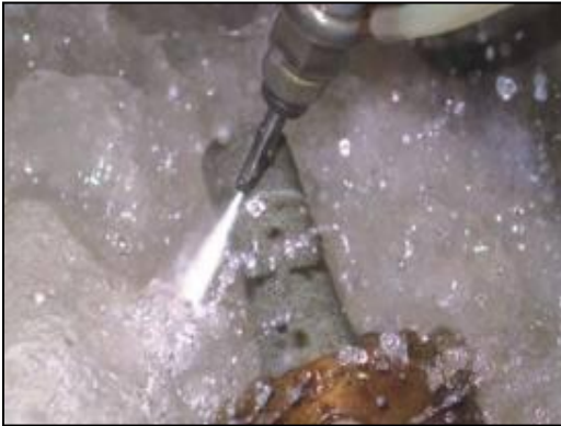
Pulsating water jet is used to break concrete
