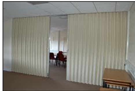
Remove partitions and combined to make a larger room
