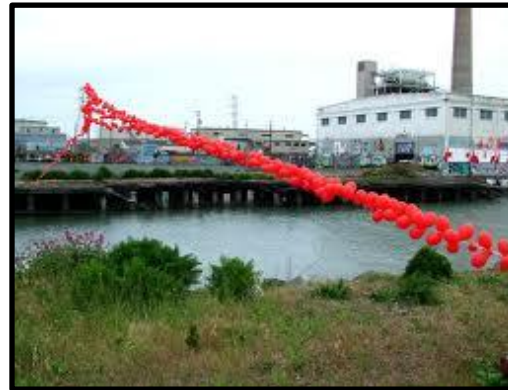
Helium balloons helps to temporarily suspend a cable over the river
